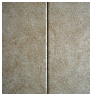
↑ Vertical wrap around finish with no vertical edge trim
